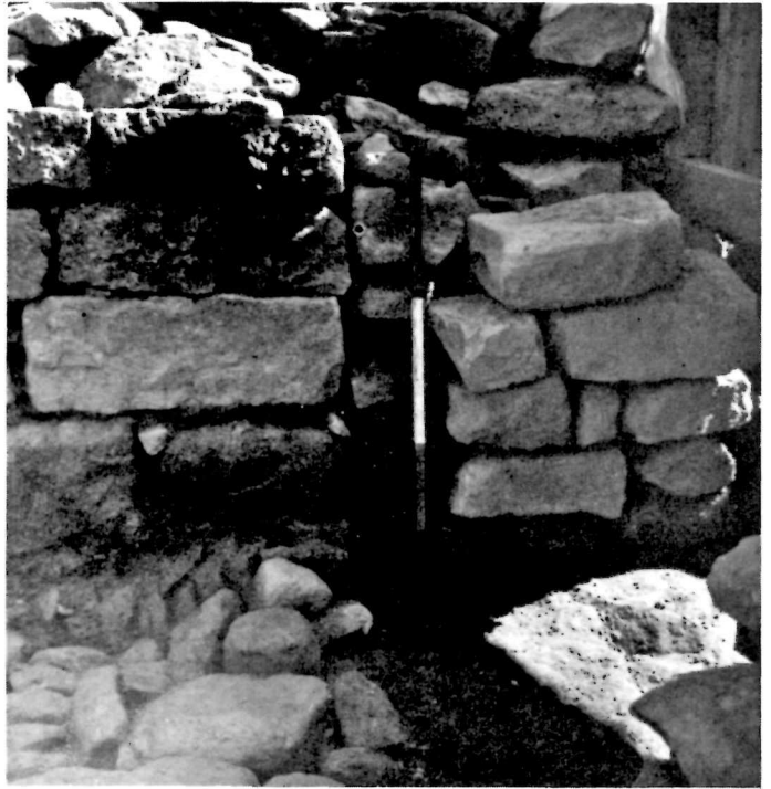
Fig. 13 - 2E20L: View of abutted joint between the north passageway wall and the well entrance. Facing North. 3' scale. (2E-586-X)
