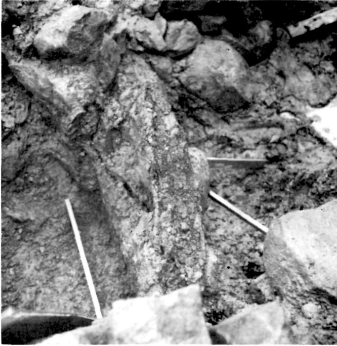
Fig. 16: (2E-697 X) The top of the door of Sill #2 on Fig. 2. The camera is facing northeast. 2' scale.
