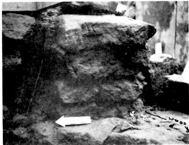
Fig. 11 - 2E20K: View of south side of well entrance showing break in the construction plus stone slot. 6" scale, Facing Southwest. (2E-137-M)
